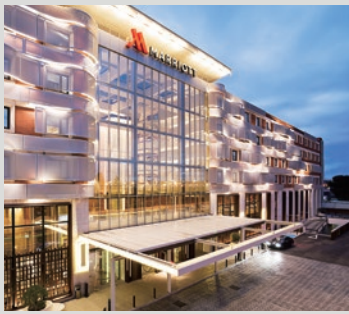
Marriott Auditorium Hotel, Madrid, Spain
